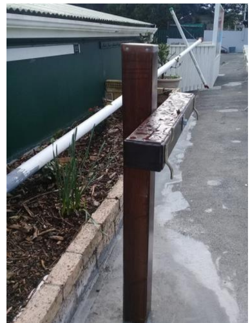
The base for the new flagpole waiting.....
